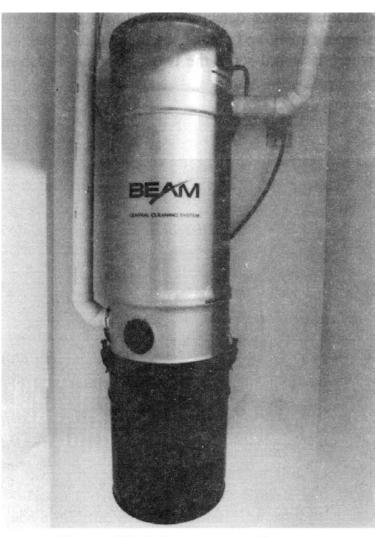
Figure 25-5. Beam central vacuum mounted in laundry closet.
