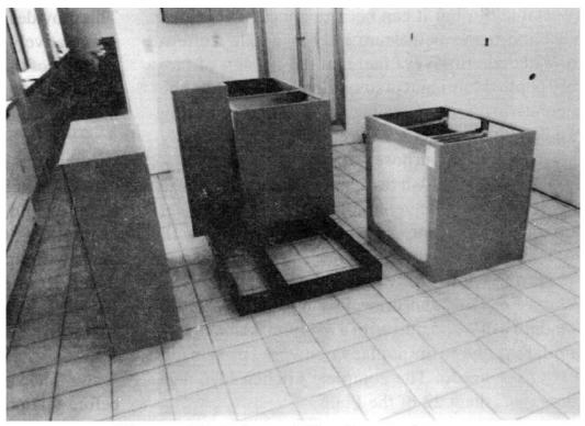
Figure 23-4. Assembling base cabinets.
