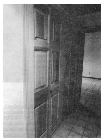
Figure 26-2. Solid wood interior bi-fold doors.
