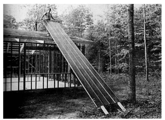
Figure 7-8. Pulling the roofing up into place.
