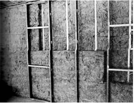
Figure 12-3. Fiberglass and steel framing.
