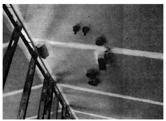
Figure 13-9. Ductwork sealed to drywall.
