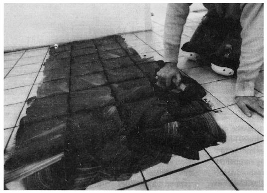
Figure 22-7. Applying grout with a rubber squeegee.
