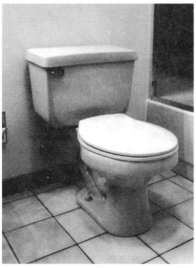
Figure 24-3. Low-flow toilet with insulated tank.
