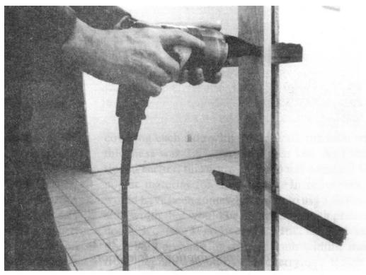
Figure 26-4. Using shims to plumb a door jamb.
