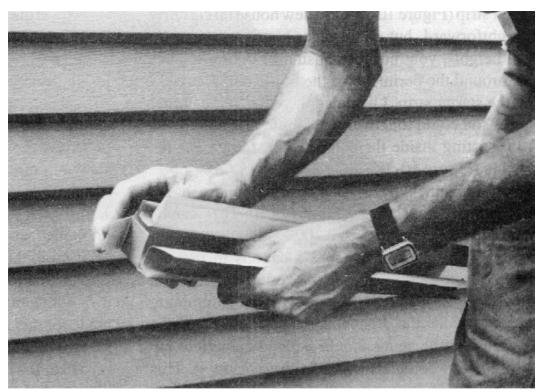
Figure 10-3. Capping the end of a corner post.
