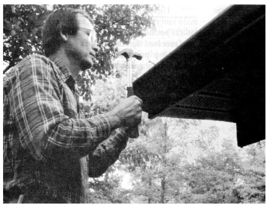
Figure 10-12. Installing gutters.
