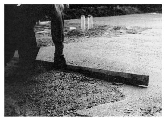
Figure 5-16. Rough leveling of the concrete floor slab.
