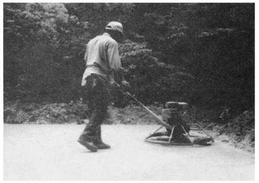
Figure 5-18. Finishing the concrete floor slab with a motorized trowel.
