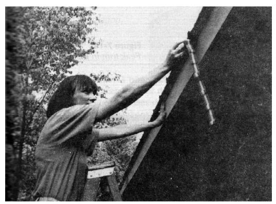
Figure 7-13. Installing foam gaskets.
