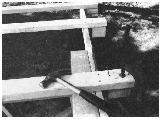
Figure 6-32. Attaching blocking at purlin ends.
