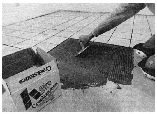
Figure 22-5. Spreading the thin-set mortar.
